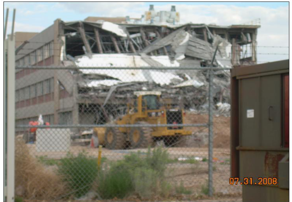
Demolition of SNL building 807 site containing high levels of toxic substances
